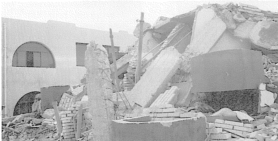
Figure 1 - Collapse of a 3-story hotel in Nuweibaa.
