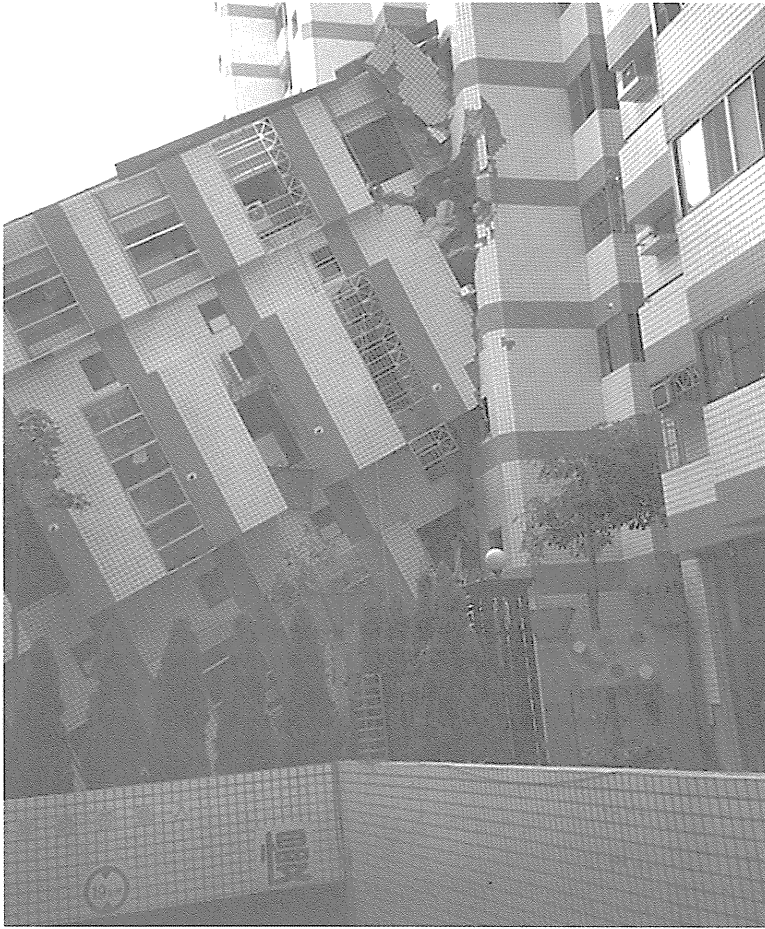
Figure 9 - Soft-story collapse of a mid-rise apartment building, Dali. (Photo: Meyer)
