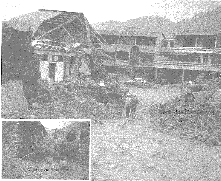
Figure 5 - Fault surface rupture at a water filtration plant near Feng-Yuan. (Photo: I.P. Lam)
