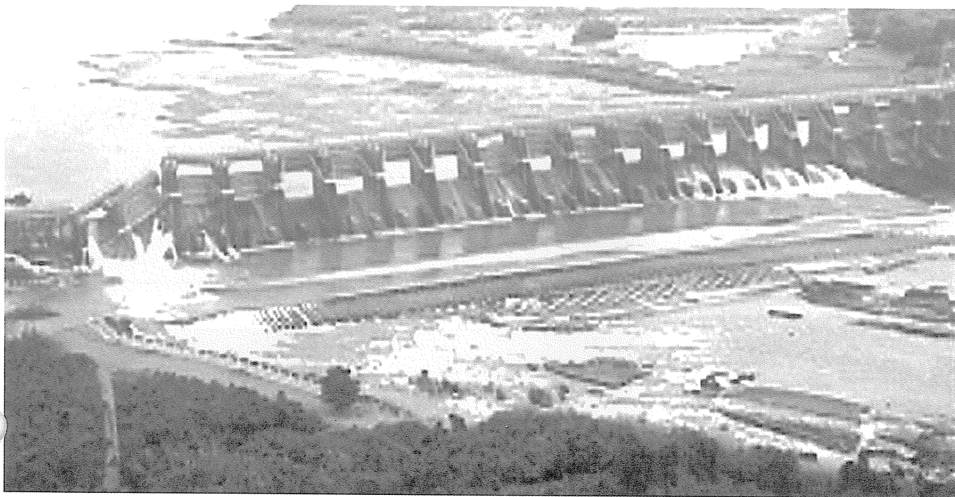
Figure 4 - Fault surface rupture across Shih-Kang Dam.
