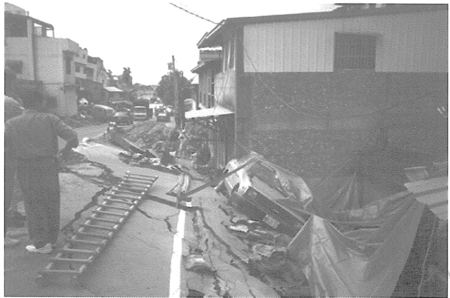
Figure 6 - Undamaged building with unreinforced brick walls immediately adjacent to fault rupture. (Photo: Uzarski)
