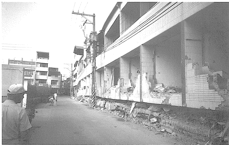
Figure 10 - Double pancake of four-story building. Only two stories remain. (Photo: Uzarski)
