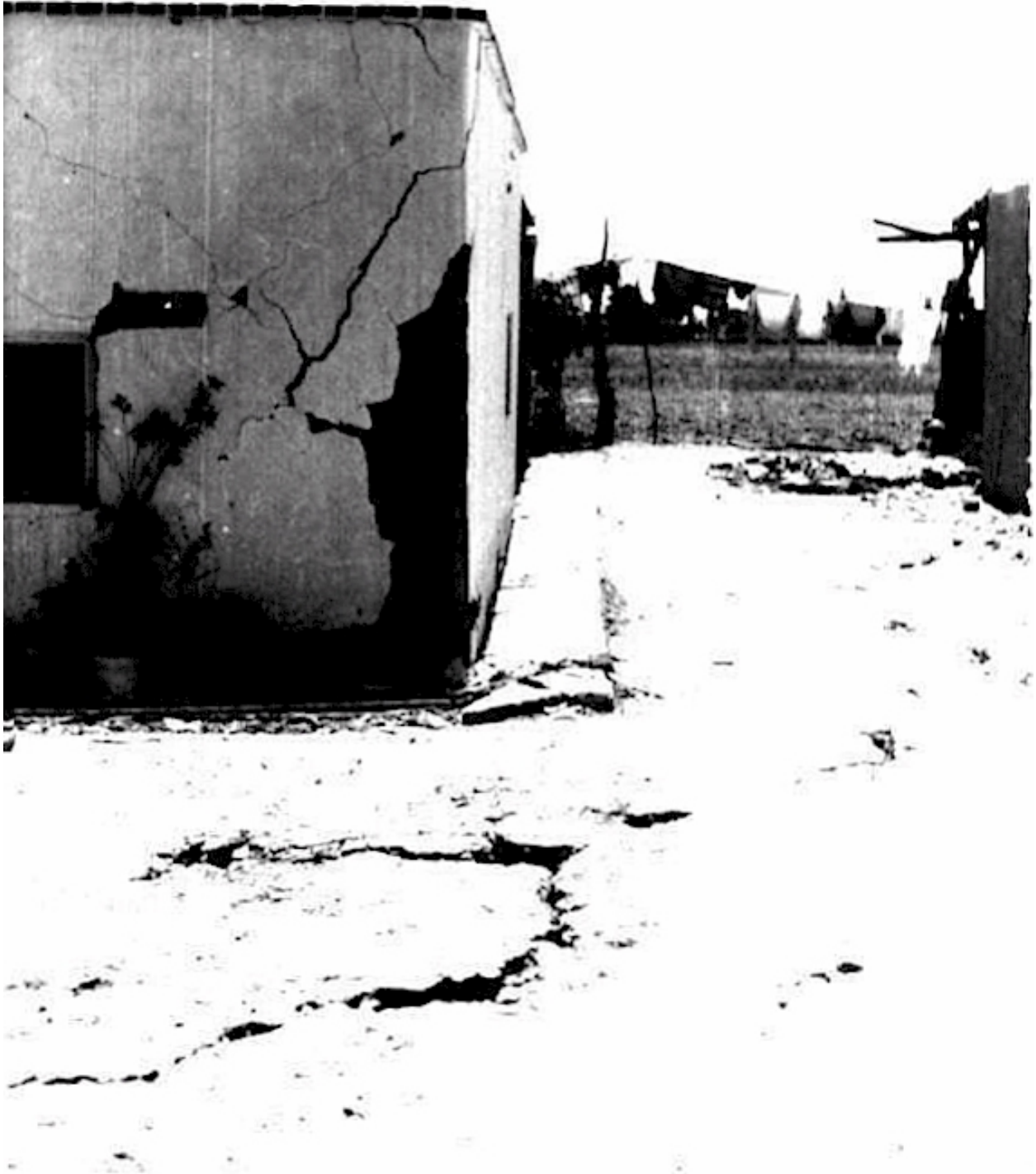
FIGURE 6A: Photograph Illustrating Typical Earthquake Damage
