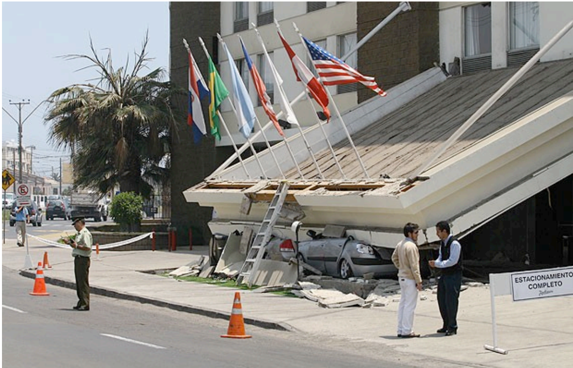
Figure 5. Roof collapse in the city of Antofagasta (Source: www.emol.com )
