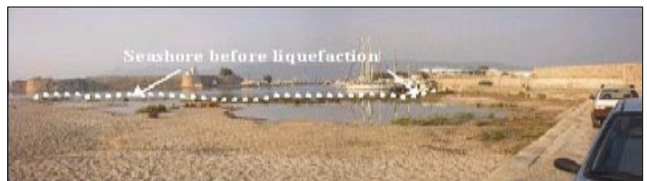
Figure 12. Area near the castle of Lefkada where soil liquefaction, lateral spreading, and ground settlement occurred (ITSAK team).
