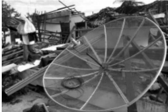
Residential damage in Bengkulu, Sumatra Island (AP Photo/Charles Dharapak).
