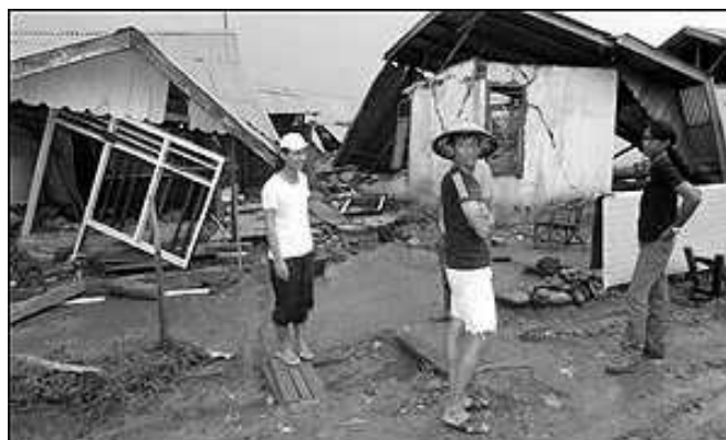
Residential damage on Enggano Island (photo: BBC News web site).
