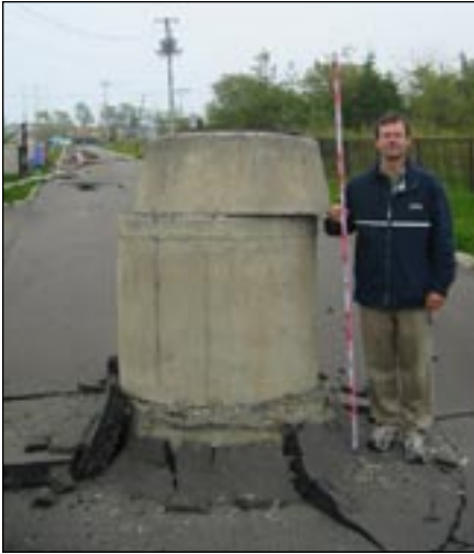
Figure 5. Uplifted manhole near sewage treatment facility in Otsu.
