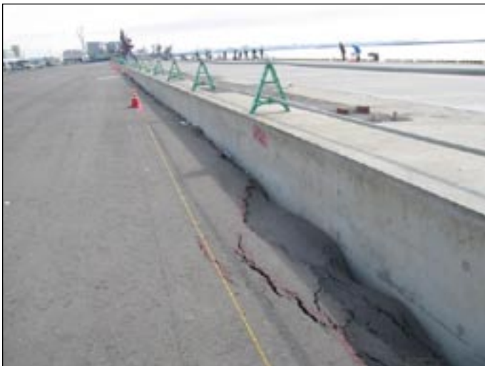
Figure 4. Pier 4, Port of Kushiro.
