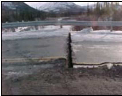
Figure 14 - Embankment movement
