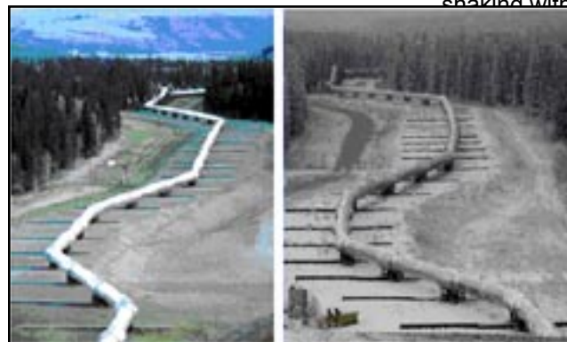
Figure 9 - Pipeline location pre-earthquake (left) and post-earthquake (right)
