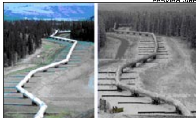
Figure 9 - Pipeline location pre-earthquake (left) and post-earthquake (right)
