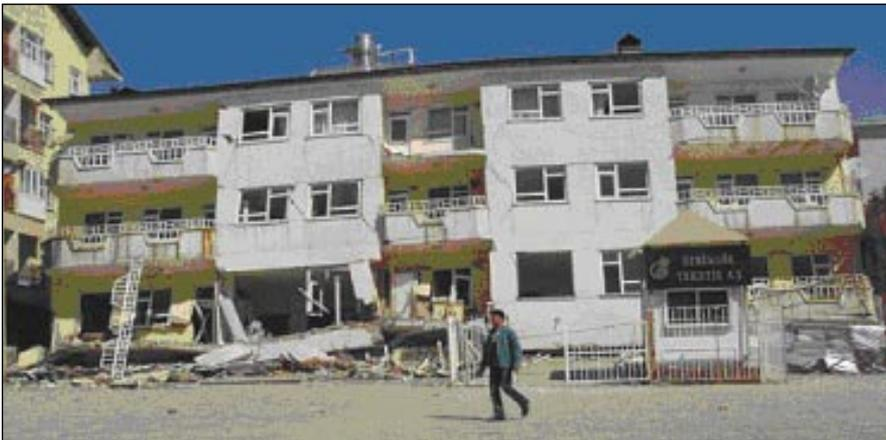
**Figure 17.** Typical first-story collapse.
