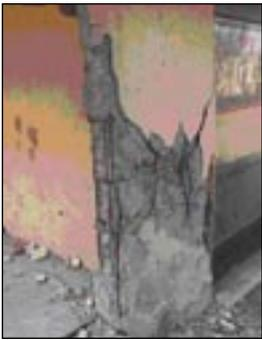
**Figure 9.** Shear failure at column base due to insufficient amount of transverse reinforcement.
