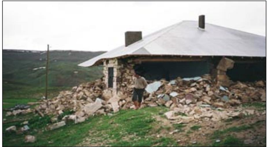
**Figure 14.** A traditionally built rural house that was heavily damaged.
