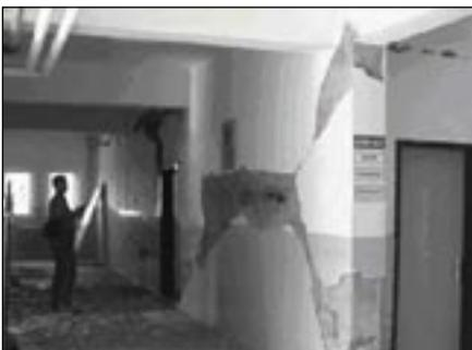
**Figure 10.** Observed shear failure at shear wall due to insufficient transverse reinforcement and poor concrete quality.
