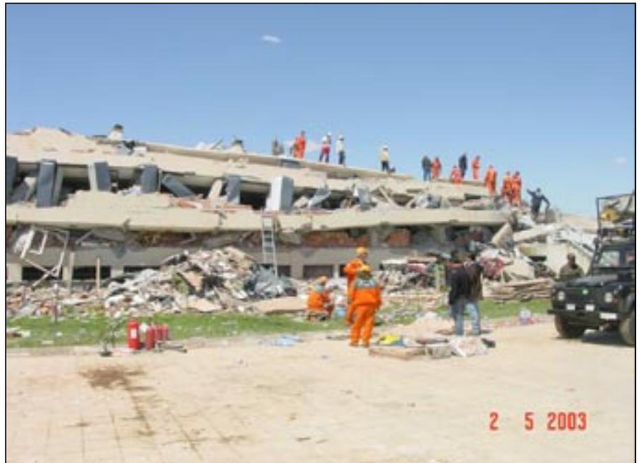
**Figure 12.** Metal storage lockers partially support floor of school.
