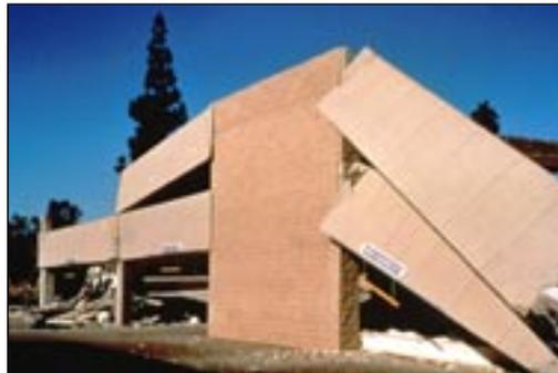
*During the Northridge earthquake, a precast concrete parking garage at the Northridge Fashion Center almost completely failed, even with little damage to some of its masonry shear walls. (Photo credit: EERI Northridge Earthquake Reconnaissance Team)*
