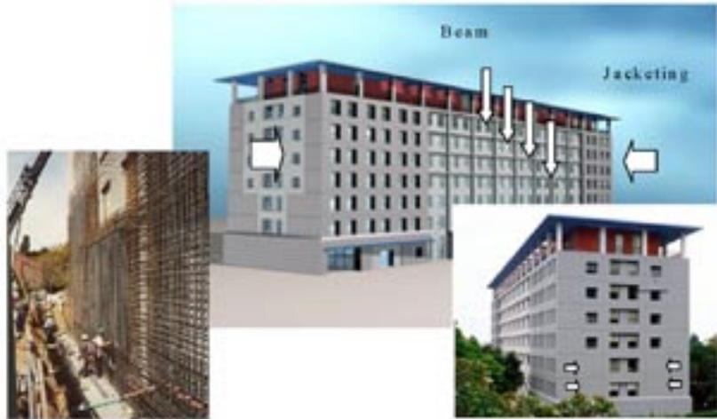
*Barrows Hall at UC Berkeley, originally completed in 1964, was retrofitted in 2002 by Degenkolb Engineers. The jacketing scheme increased the strength and stiffness of the building by adding shear walls at the ends and allowed the building to remain inhabited during the construction process.*
