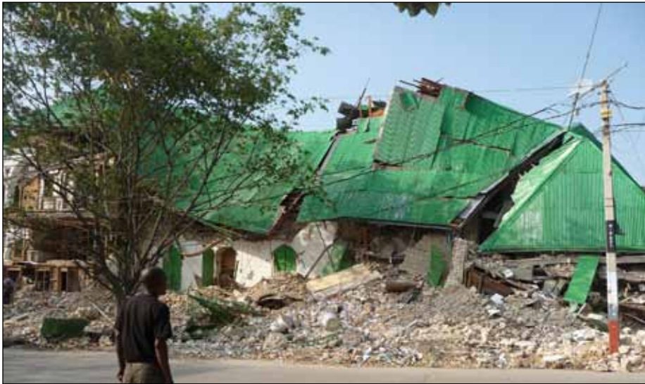
Figure 5. Unreinforced masonry Ministry of Interior building (photo: Martin Hammer).
