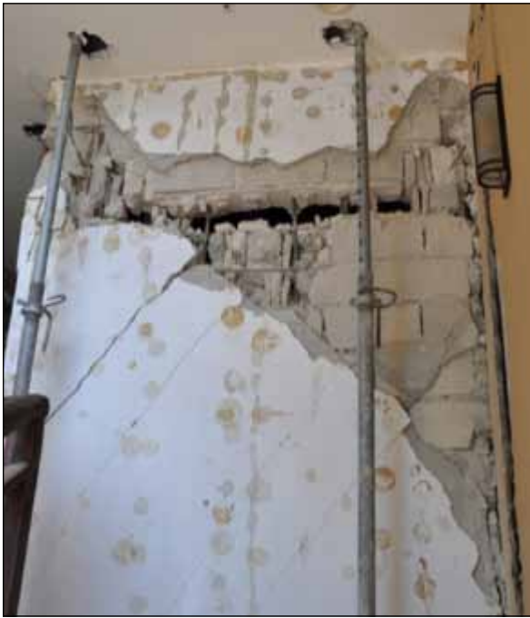
Figure 8. Reinforced CMU wall from a hotel in Petionville (photo: Amanda Lewis).
