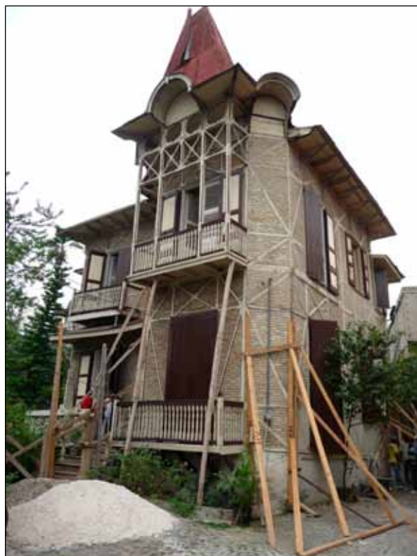
Figure 2. Timber frame with colombage (photo: Martin Hammer).
