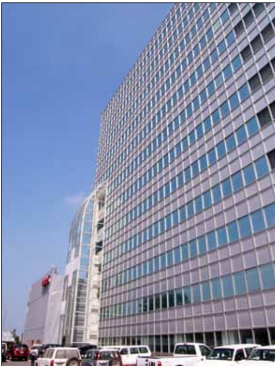
Figure 7. The 12-story Digicel building with RC dual (frame-wall) structural system (photo: Anna Lang).
