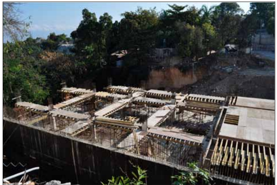
Figure 10. Garage of hotel under construction, sustained no damage (photo: Ayhan Irfanoglu)
