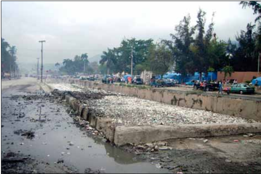
Figure 18. Sediment and debris (mostly plastic bottles) build-up in drainage channel at highway overcrossing (photo: Anna Lang)
