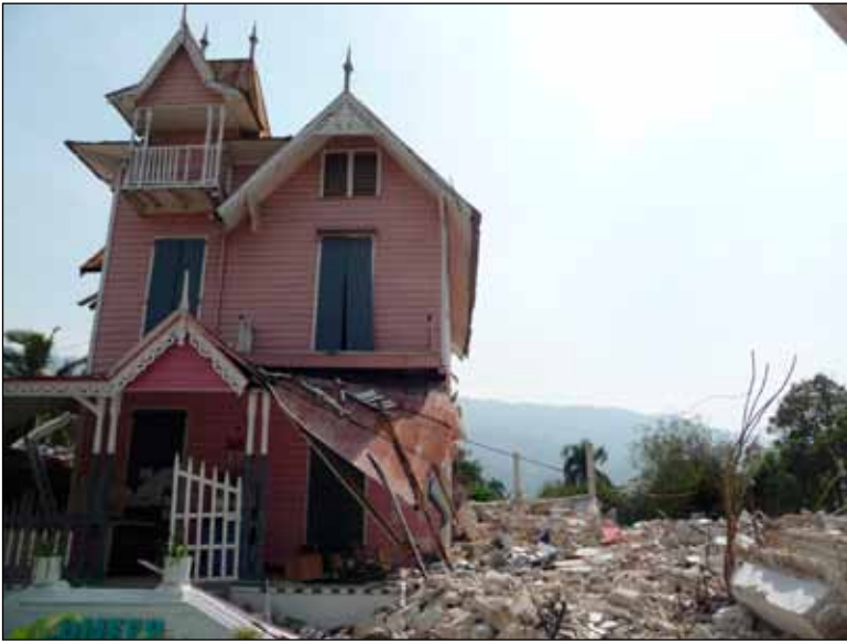
Figure 3. Wood frame building next to collapsed concrete and masonry building (photo: Martin Hammer).
