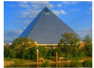
The Memphis Pyramid: One of the largest seismic retrofit projects in the eastern U.S. (photo: Exo-thermic)
