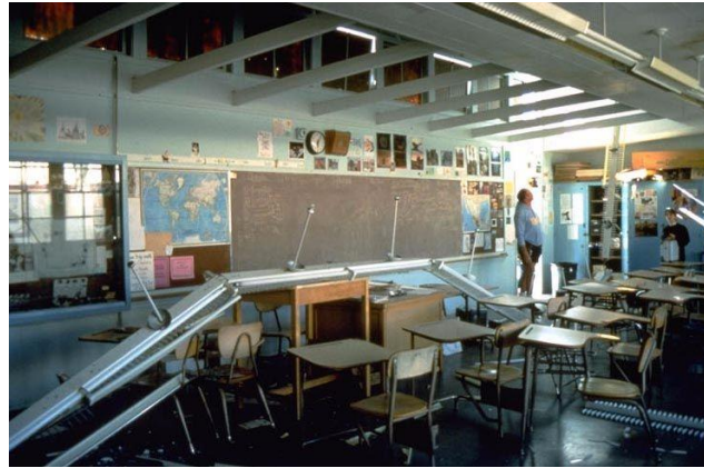
Fig. 8 – Lights fell onto desks in a Northridge Junior High classroom during the 1994 earthquake. School was not in session, so no injuries occurred (photo: Gary L. McGavin) [19].
