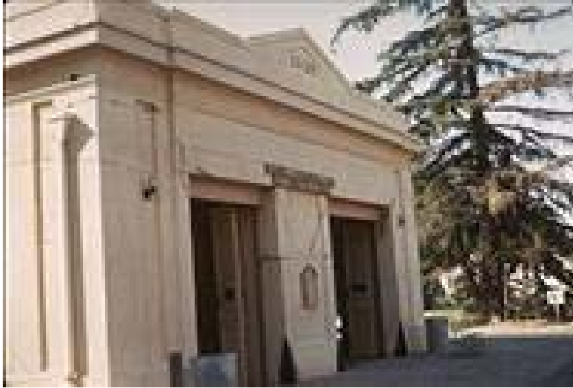
Fire station at Olive View Hospital damaged in the 1971 San Fernando, California earthquake
