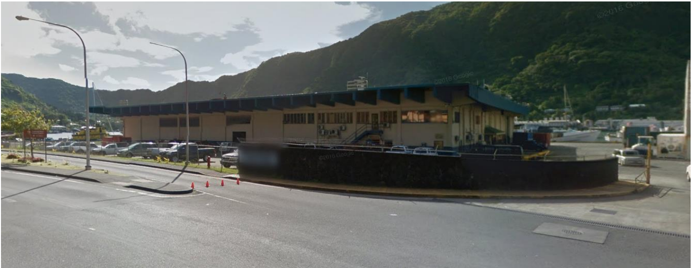
Figure 3. Street view of Optional Building A
