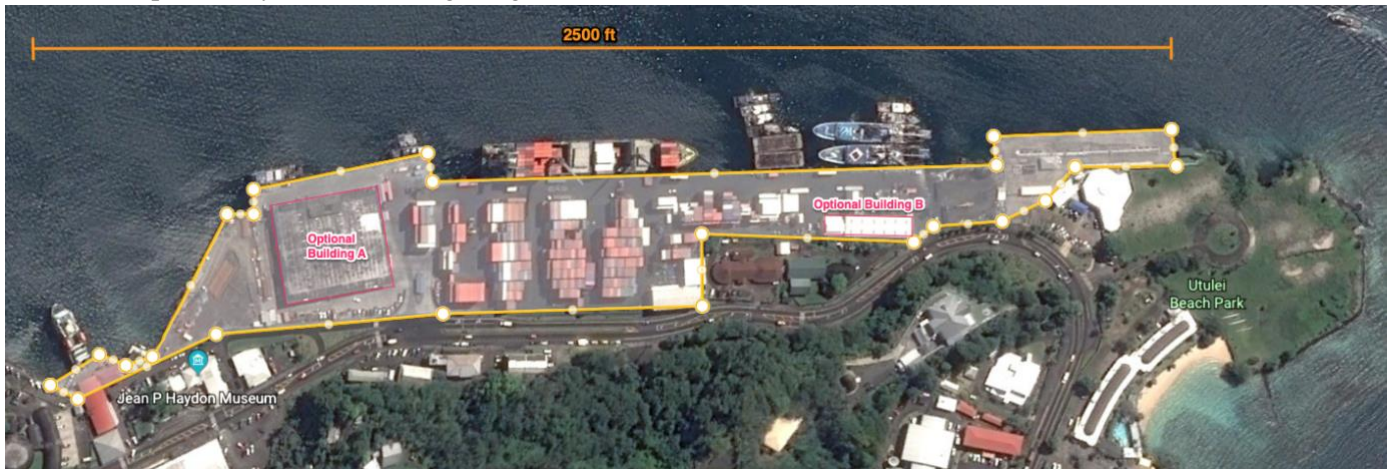
Figure 1. Approximate outline of the wharf area to be assessed is outlined in yellow. The wharf is approximately 525,000 square feet in area and 2500 ft in length. Optional Buildings A and B are shown in pink. To explore the wharf in Google Earth, please visit https://earth.app.goo.gl/RyMW2x .
