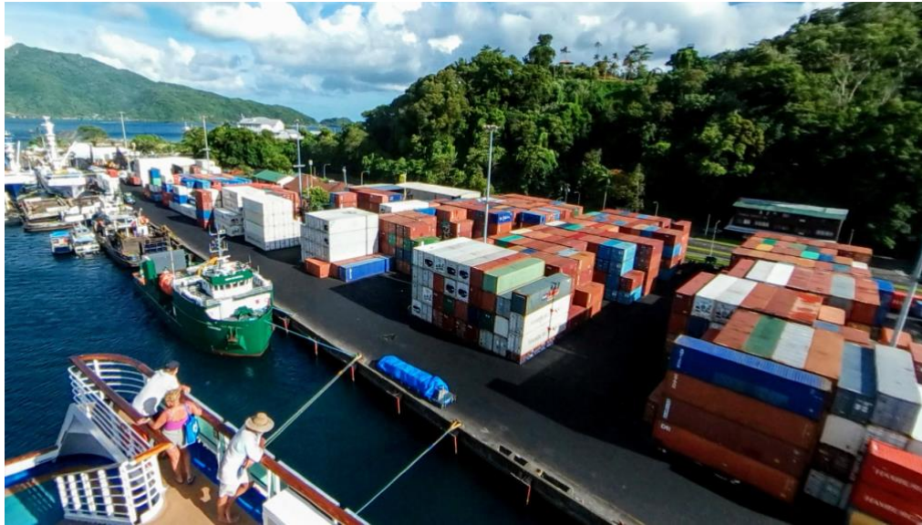
Figure 2. View of wharf structure from a moored cruise ship.
