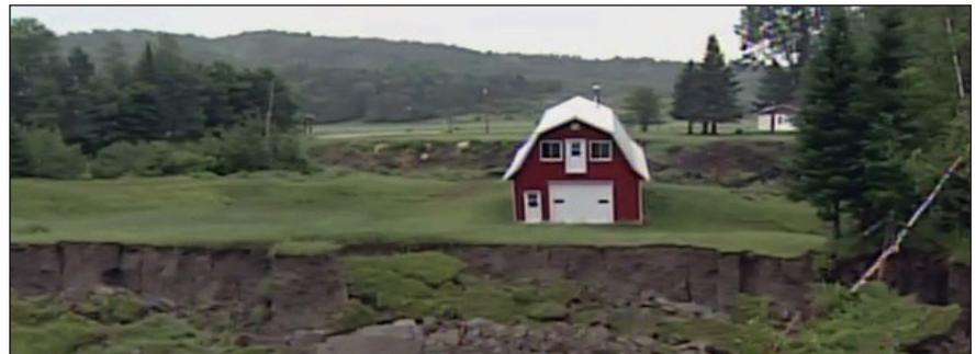
Landslide near the epicenter resulted in 50 m of downhill movement, soil failure, and damage to a barn foundation near Gracefield, close to epicenter.
