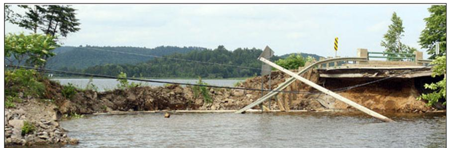
Embankment failure south of Bowman, Quebec (photo: Jean Levac).
