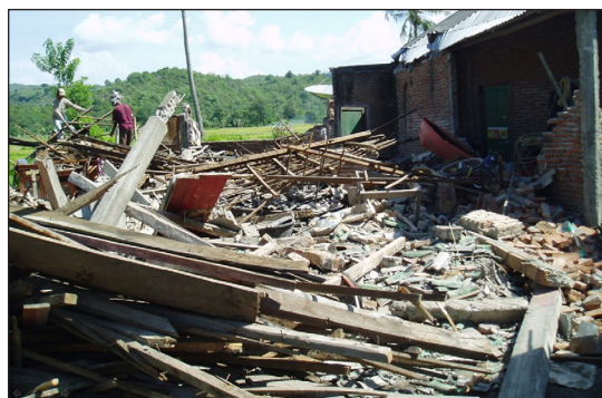
Collapsed building on Sumbawa Island (photo: Teddy Boen).
