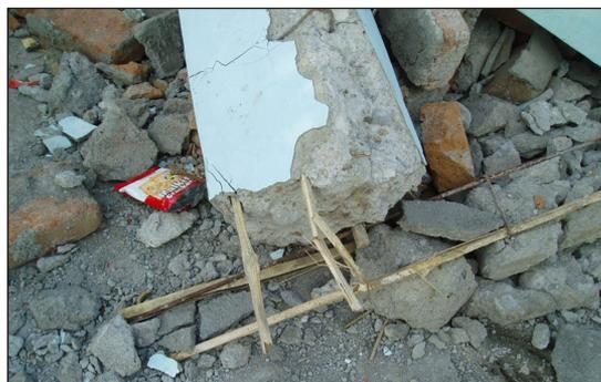
*Poor joint detailing on collapsed building (photo: Teddy Boen).*
