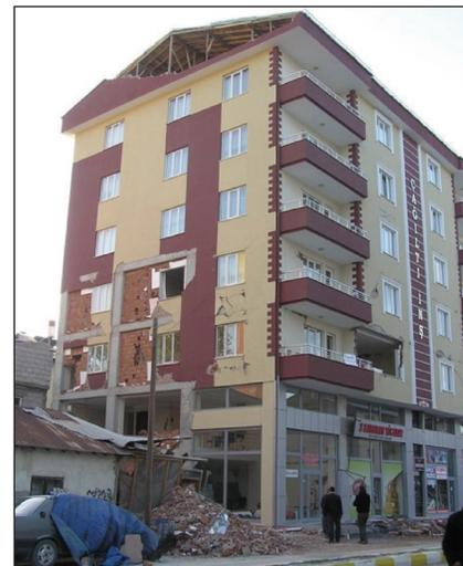
**Figure 2.** A newer building in Ercis with a typical tall ground story and mezzanine level for commercial use (photo: A. Irfanoglu).
