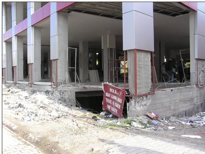
**Figure 1.** A heavily damaged six-story building in Ercis. The structural layout resulted in excessive floor torsion. The flexible joist floors with block infills had cracks around columns at every floor level. The columns failed at the base of the ground story (photo: A. Irfanoglu).
