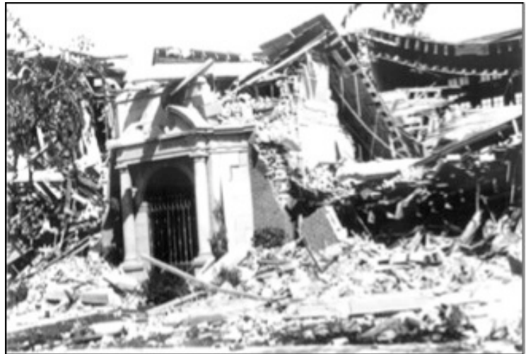
Jefferson Junior High School in Long Beach, California, destroyed by the March 11, 1933, earthquake (source: USGS, 1993).
