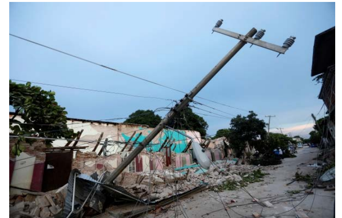
Damaged power line in Juchitan (Photo - Reuters)
